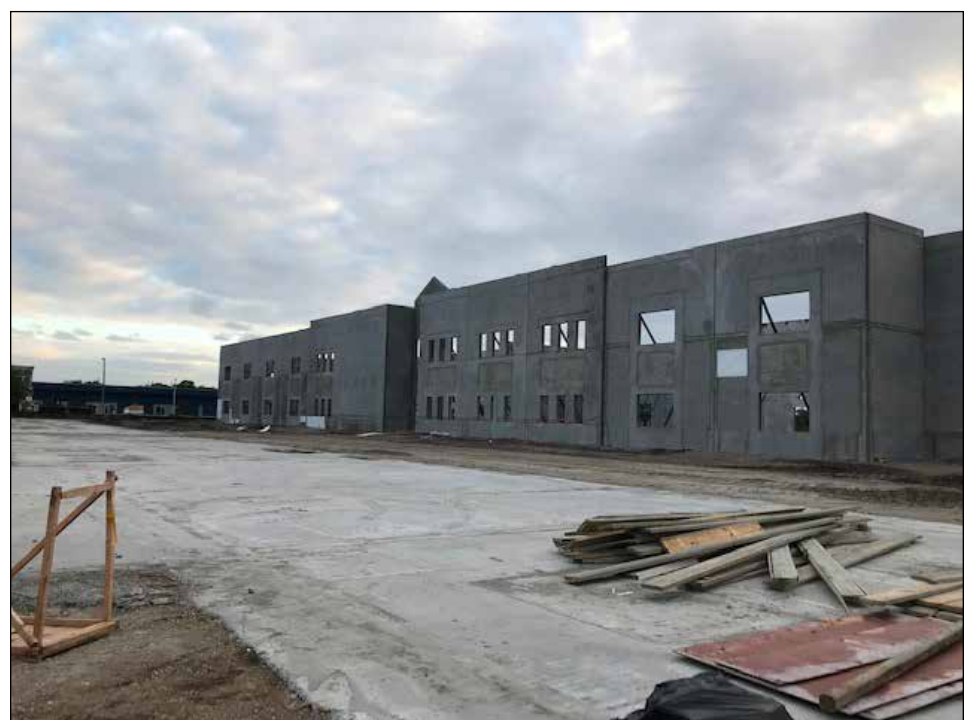
Gloomy day, but bright future! CIJS construction site, photo by Elaine Vail.
